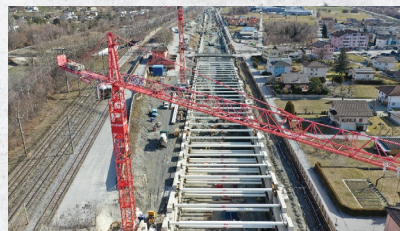
A9 Tagbautunnel – Raron (CH)
